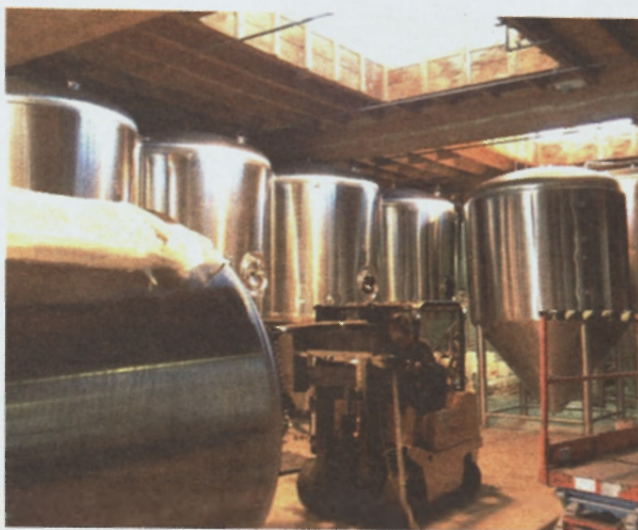
Mission Brewery forklifting in their new 90-barrel fermentation tanks. Photo courtesy of Mission Brewery
