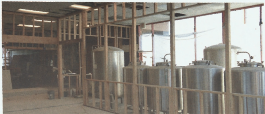
Fermenters temporarily housed in the future conference/party room
