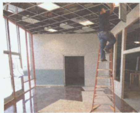
Electrical going in at ECBC
