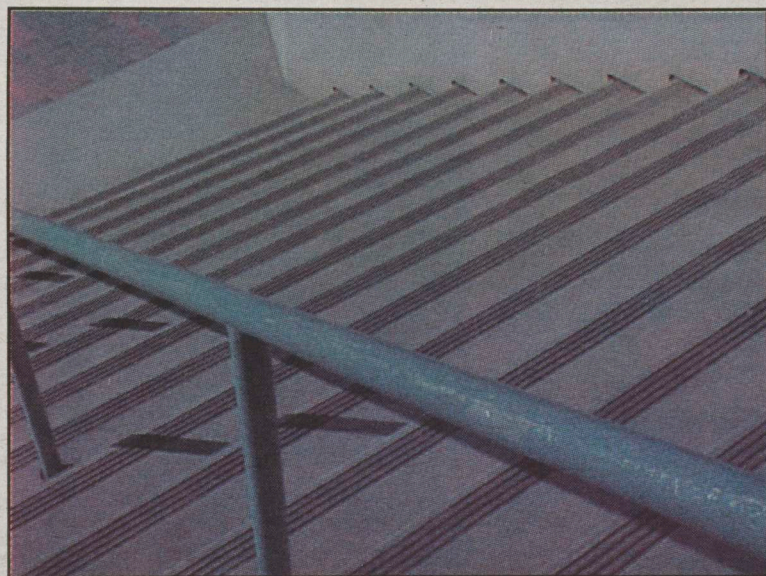
Damage to railing from skate boarding. Photo by Jennifer Jarrell
